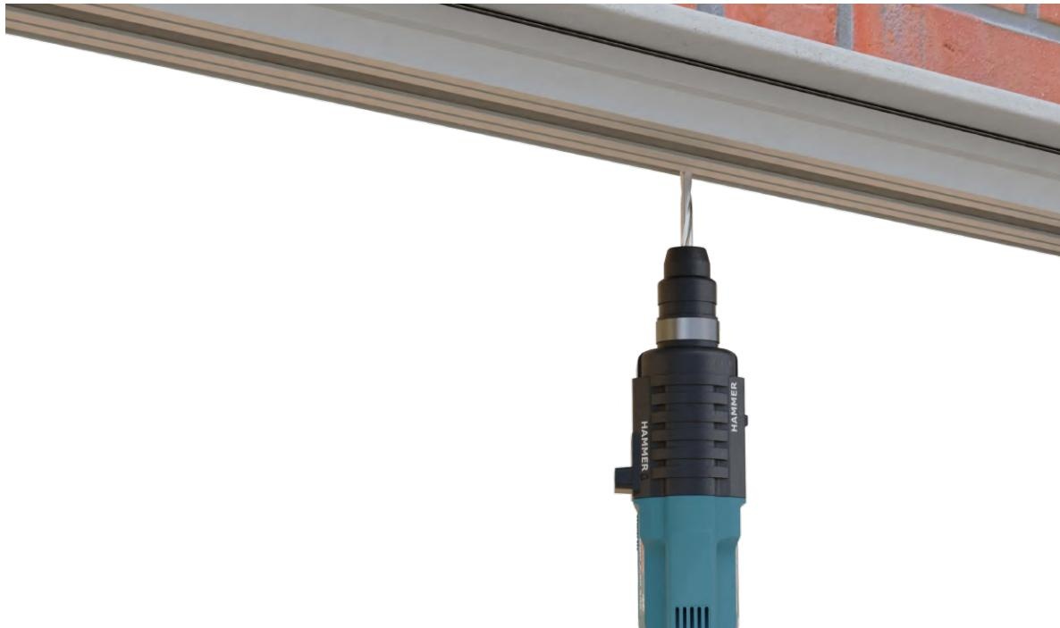
**15** Drill and countersink an appropriate sized fixing hole through the frame. This should be no more than 200 mm from the external corner of the frame.
