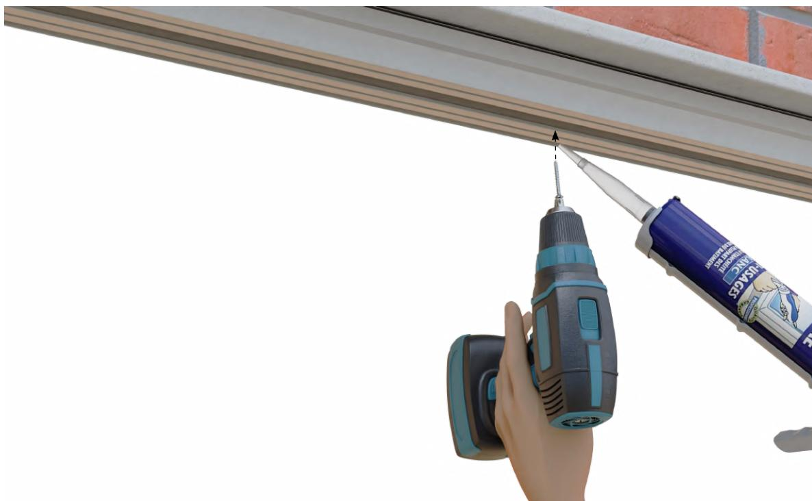
**16** Insert suitable sealant to fixing hole, then screw preferred fixing in place. Repeat process along the bottom track, ensuring fixings are within 900 mm intervals.
